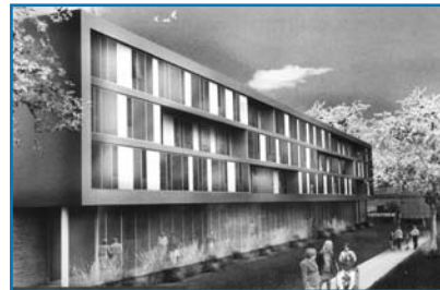
Reena Community Residence under construction on the Lebovic Campus
