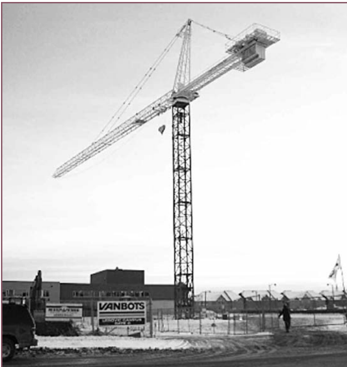
Crane installed January 6, 2011
