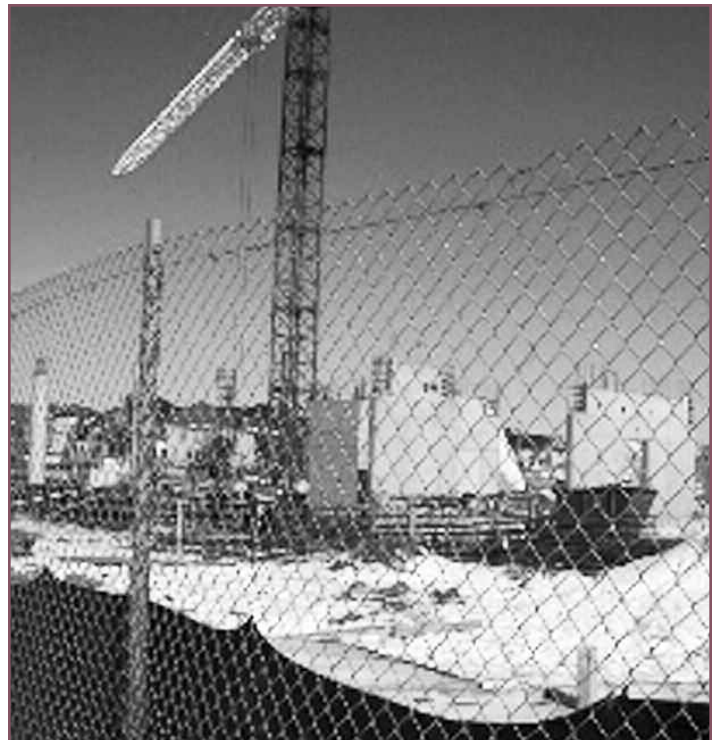
Footings in place February 21st, 2011
