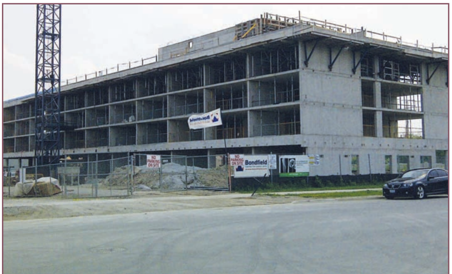
June 9, 2011 – Final floor capped off.
